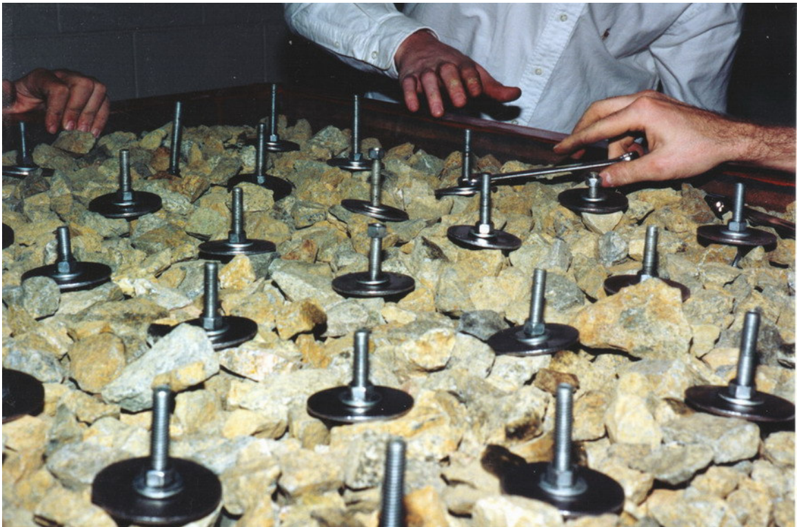
Figure 11: Washers and nuts placed on the rockbolts and tightened.
